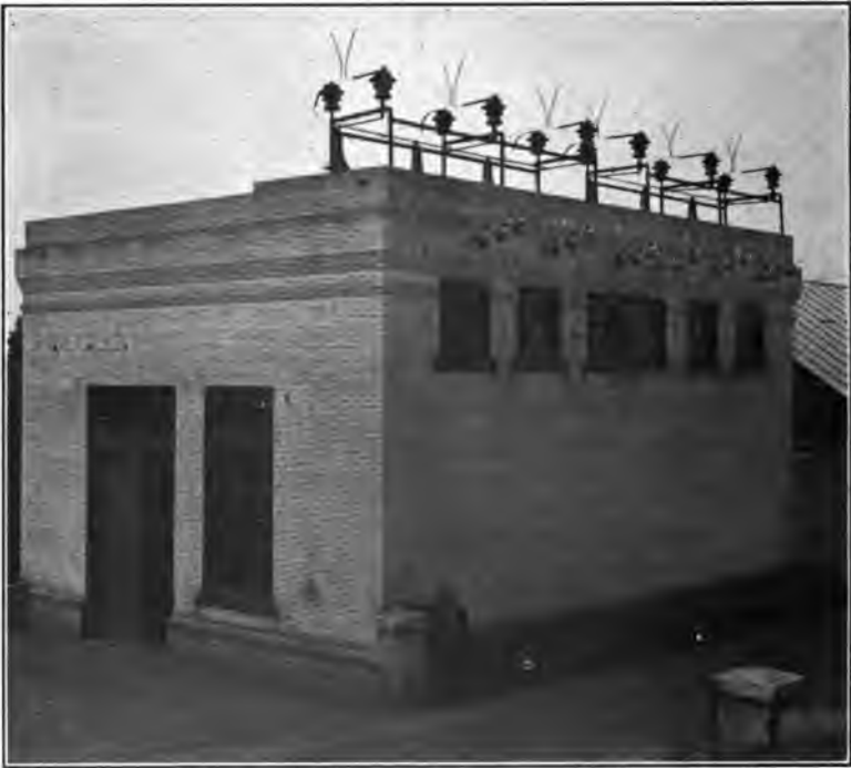
ONE OF THE SUB-STATIONS, NORTH LAKE. OUTSIDE MOUNTING. LIGHTNING ARRESTERS
